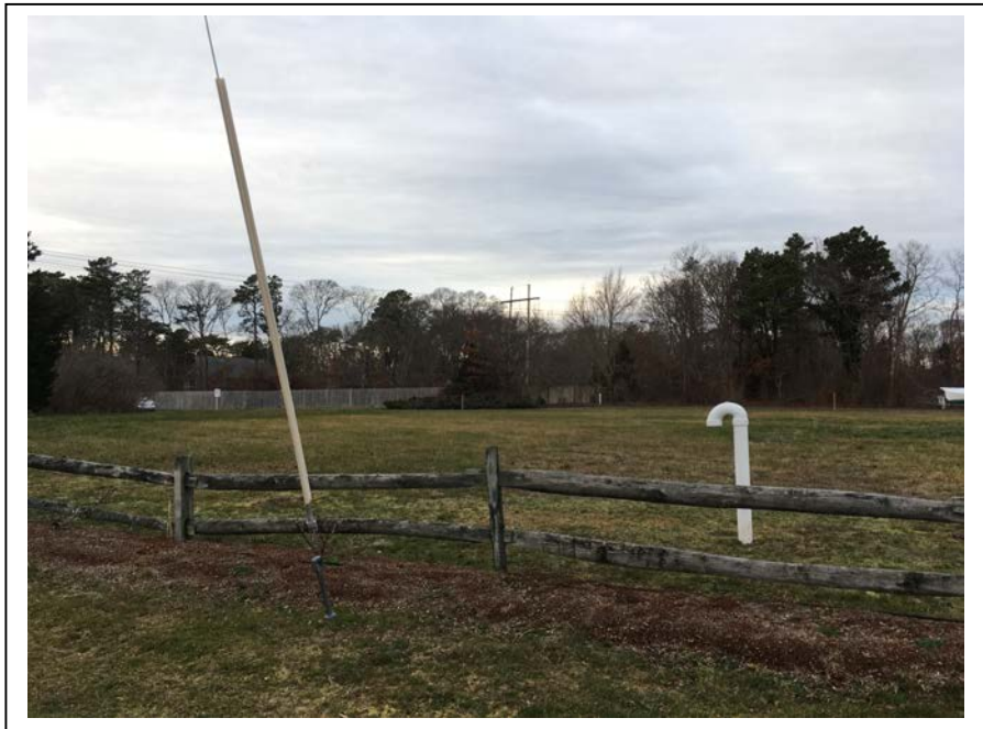
Photograph 6. Pump Station #1, Old Colony Way, view northwest.
