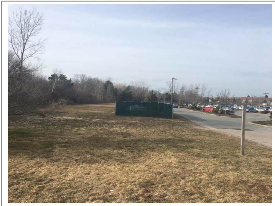
Photograph 8. Pump Station #3, view north.
