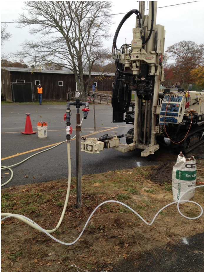
Figure 4: Direct-Push Injection Point and Geoprobe
