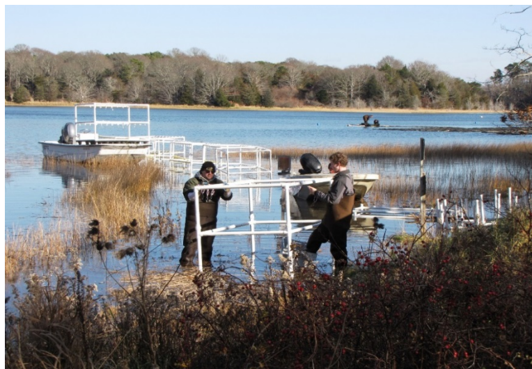
Figure 23 - Staging of Overwintering System for Installation
