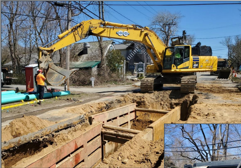
Excavator and Shoring
