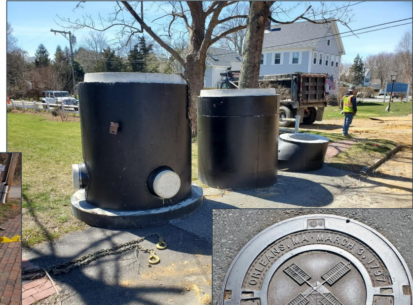
Buried and Surface Manhole Components
