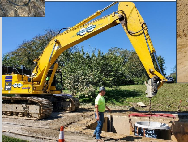
Setting a Manhole on School Rd
