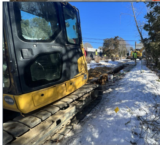
Mini-Excavator on Bayberry Way
