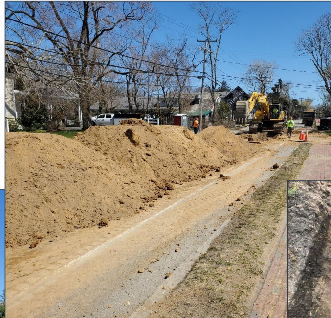
Staging the Spoils on Main St
