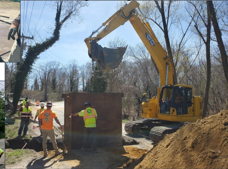
Setting Shoring for a Lateral
