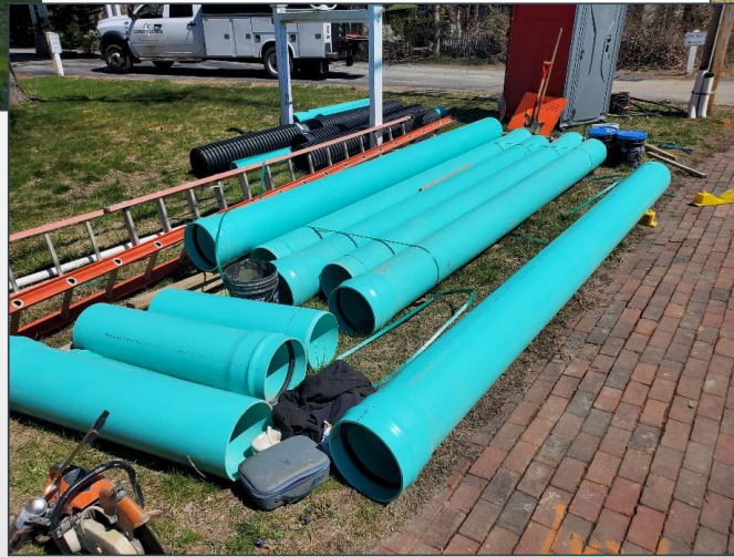
12" Gravity Main on Main St
