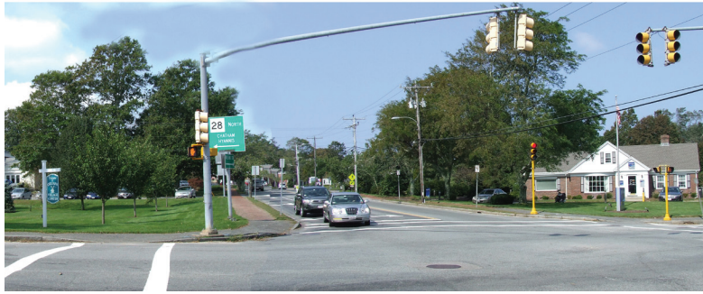
Existing: View West at 28/Main Street
