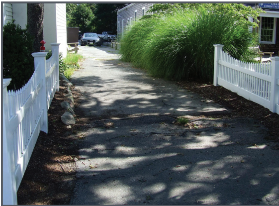
Existing: Looking North at pedestrian connection
