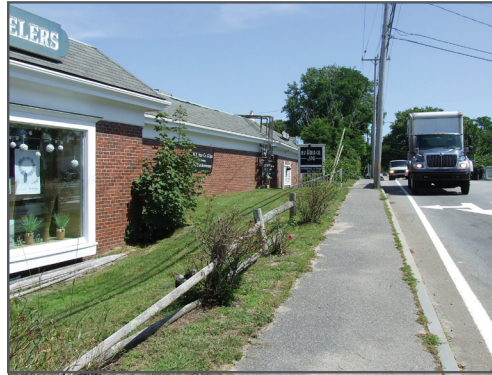
Existing: Looking North along west side of Route 6A
