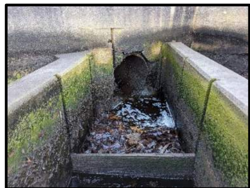
Photo 11: 30-inch Culvert beneath Herring Run Way
