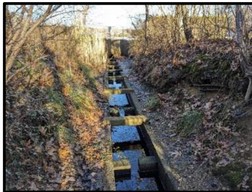
Photo 3: Technical Fishway looking north toward Herring Brook Way
