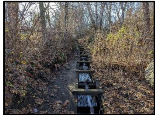
Photo 2: Technical Fishway looking south
