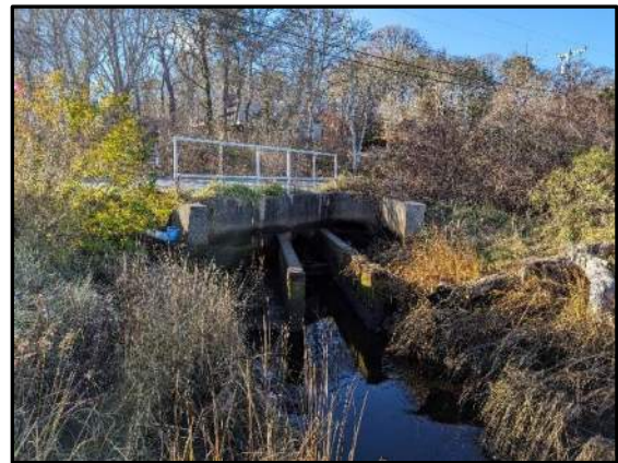
Photo 1: Herring Brook Way, fishway entrance looking south
