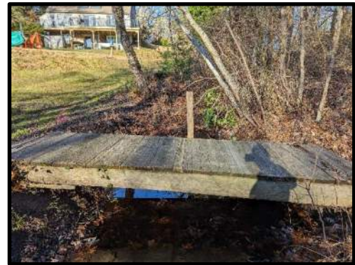
Photo 9: Example of unformalized stream crossing, Sta. 5+50
