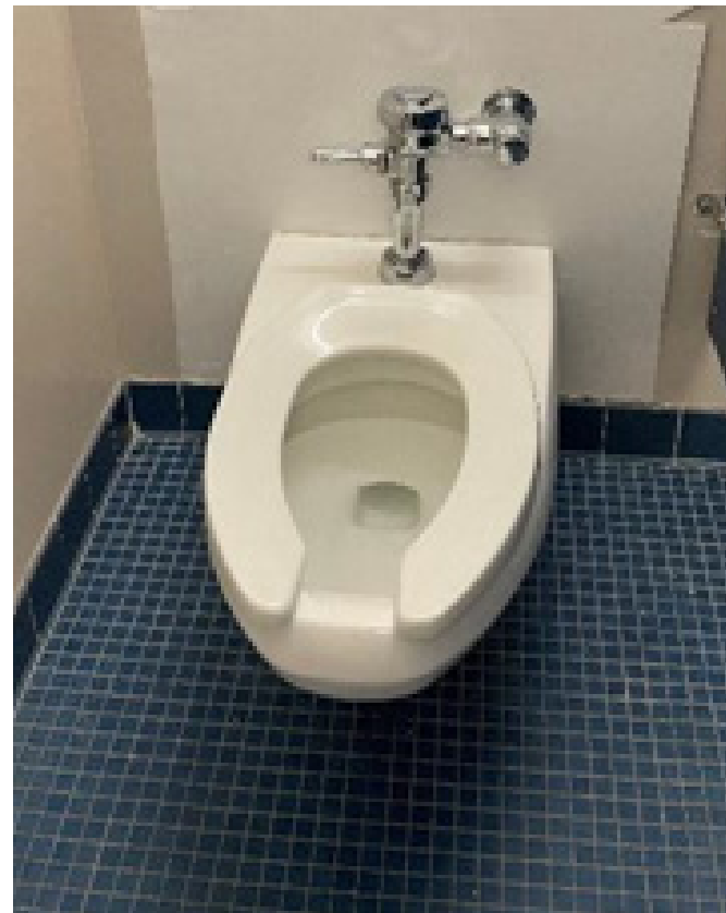
Existing Water Closet
