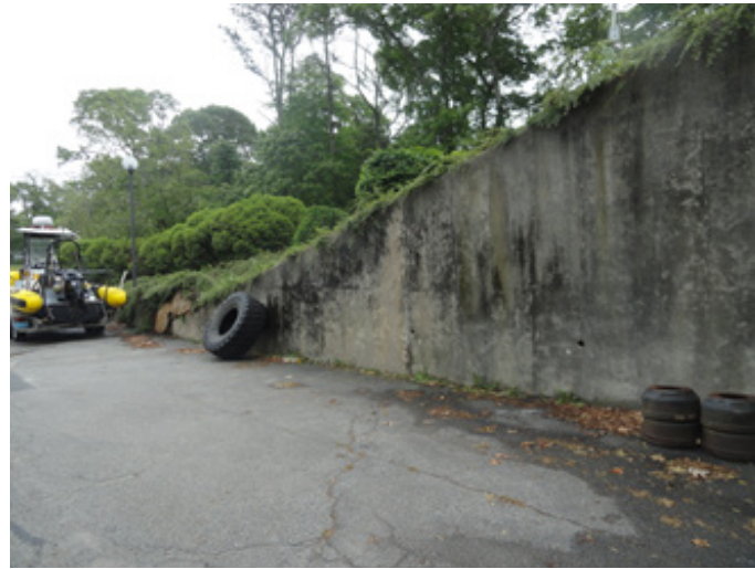
Photo #9 South Retaining Wall
