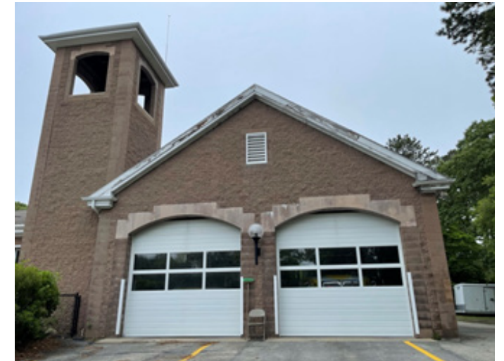
Photo #6 Building East Elevation Rescue Vehicle Garage Doors are at the 1st floor near the northeast corner
