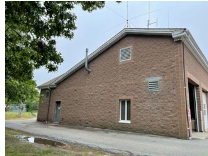
Photo #5 Building North Elevation
