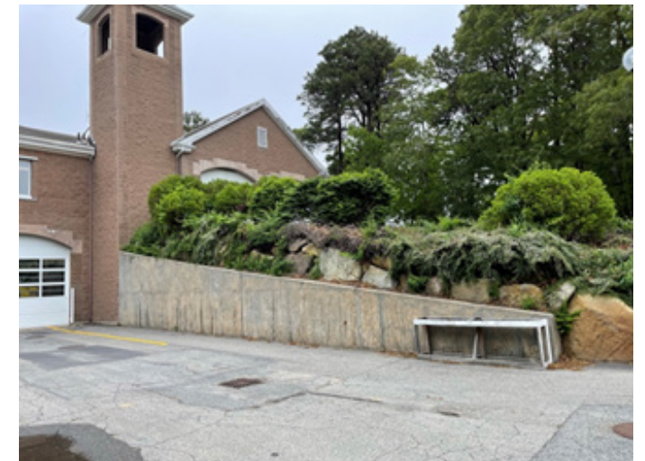
Photo #8 North Retaining Wall
