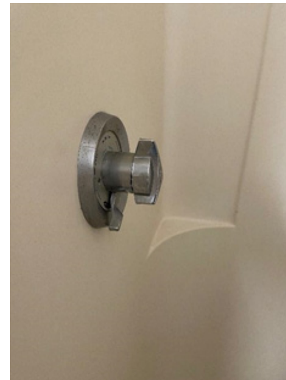
Existing Shower Valve
