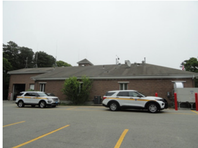
Photo #2 Building West Elevation
