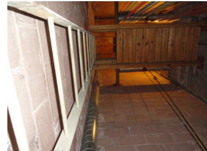
Photo #16 Hose Tower - interior masonry
