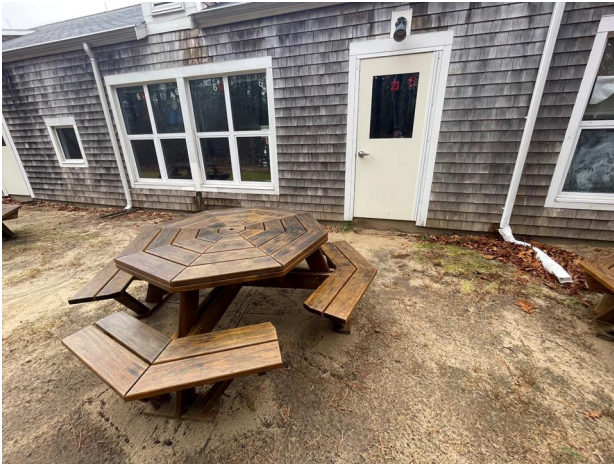
7. Topsoil is eroded and classroom doors are not MAAB accessible to outdoors.
