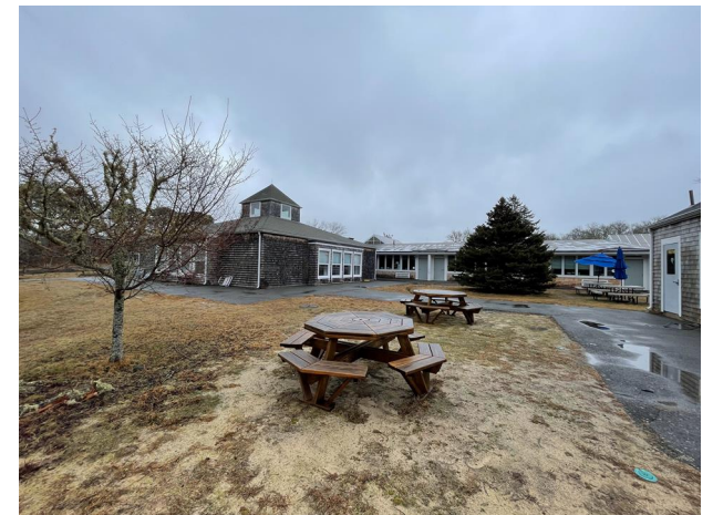
6. Topsoil in many areas is eroded.
