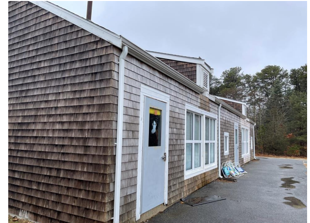
18. Hollow metal door has rust and oxidized paint. Wood fascia is peeling.
