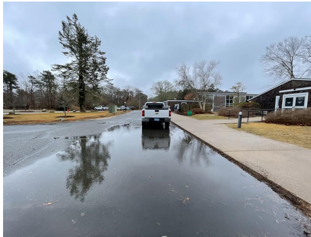
11. Large puddle in driveway.
