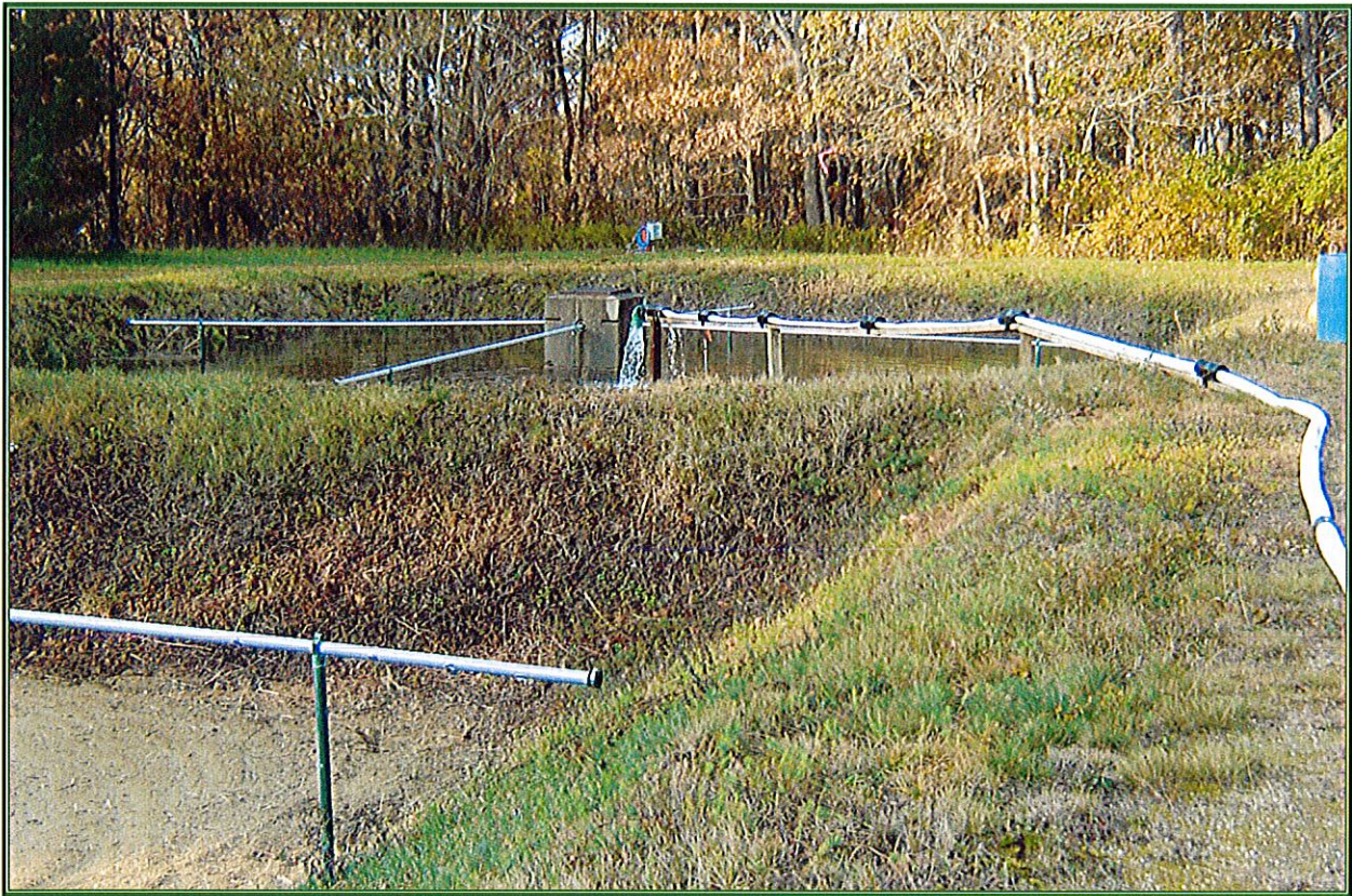
Figure 2 View of RIB No. 2 During the Operation of the Loading Test
