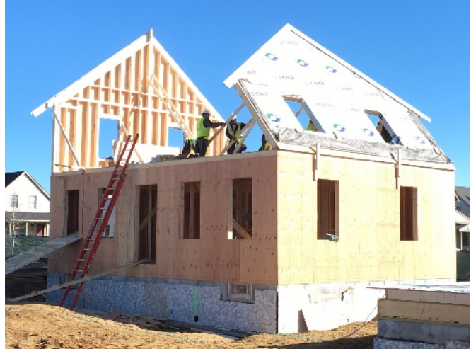
Sachem's Path, Nantucket – Under construction
