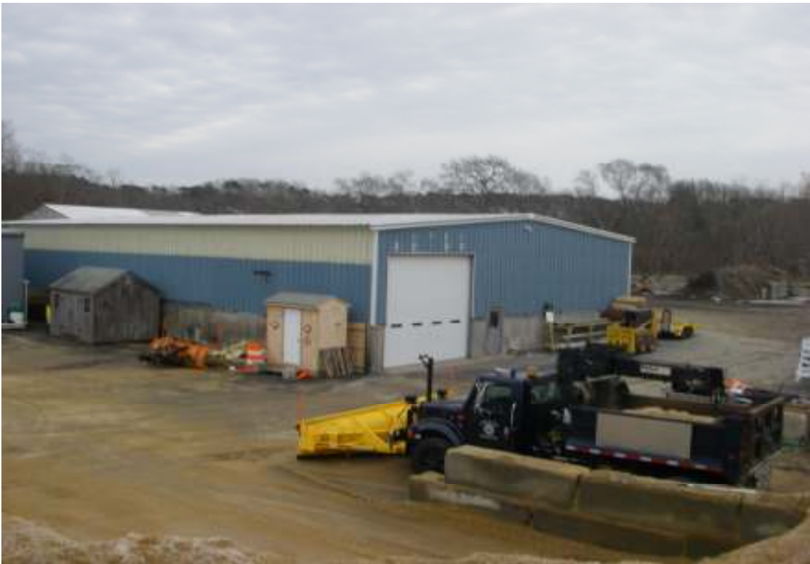
Photograph 6: Southeasterly view of Orleans Highway Department property off Bay Ridge Lane.*
