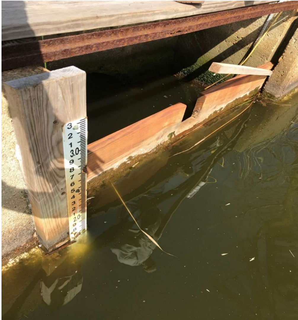
Figure III-1. Notched Board at Cedar Pond Outlet. After reviewing 2018 water levels at the outlet, Town, MassDMF, and CSP/SMAST staff agreed that the boards at the outlet could have a notch in the upper board to facilitate fish passage while also trying to limit the volume of high tides reaching Cedar Pond. Subsequent water level monitoring in 2019 showed this decreased salinity in the pond, but once it was added, salinity levels increased at the same rate as in 2018. 2020 monitoring suggested that the elevation of the bottom of the notch could be increased while also attaining similar frequency of water levels meeting the Fishway Plan goals. Notch elevations are adjusted according to Fishway Plan goals for 6 inches of water over the notch bottom in the spring for spawning herring immigration (March 15 to June 30) and 2 inches of water over the notch bottom in mid/late summer to allow young of the year emigration (July 1 to November 15). No herring have been observed during more than 81 visits from 2018 through 2021.
