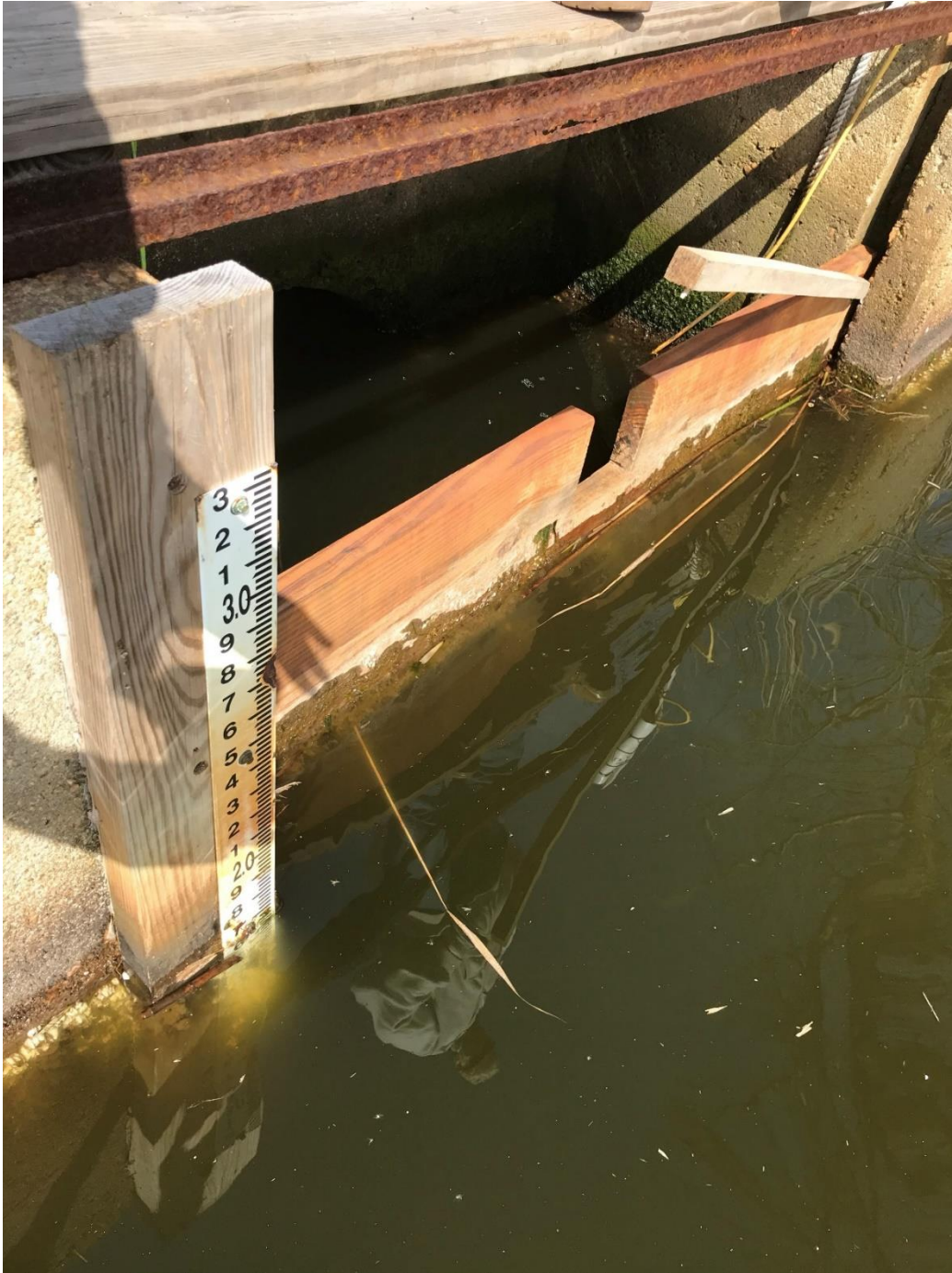
Figure III-1. Notched Board at Cedar Pond Outlet. After reviewing 2018 water levels at the outlet, Town, MassDMF, and CSP/SMASST staff agreed that the boards at the outlet should have a notch in the upper board to facilitate fish passage while also limiting the number of high tides reaching Cedar Pond. Subsequent water level monitoring in 2019 showed this decreased salinity in the pond, while 2020 monitoring suggested that the board elevation could be increased without significantly altering the number high tides reaching the pond. Notch elevation is adjusted according to MassDMF goals for high tide elevation over the notch in the spring for spawning herring immigration and a reduced elevation over the notch in mid/late summer to allow young of the year emigration. No herring have been observed at the boards in more than 30 visits between 2018 and 2020.
