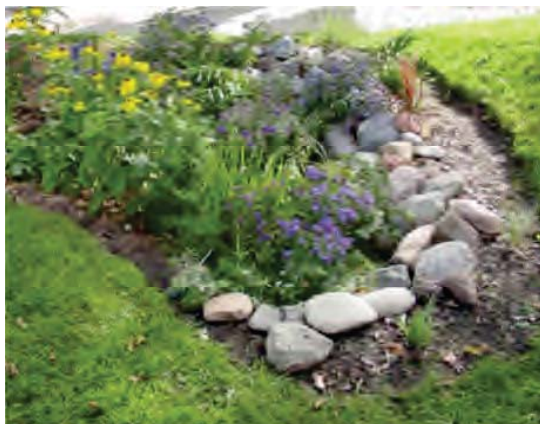
Source: Massachusetts Stormwater Handbook Figure 5-2. Bioretention area, or rain garden, on a residential property.
