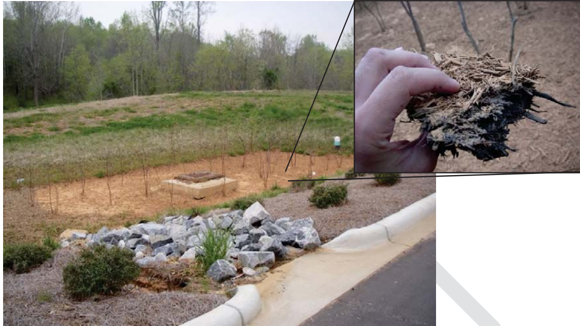
Figure 5-11. Example of a bioretention area installed before permanent site stabilization with the inset photo showing the clay layer clogging the mulch surface.
