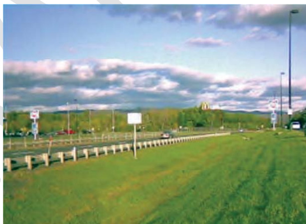
Source: Massachusetts Stormwater Handbook Figure 5-7. Water quality swale adjacent to a highway.
