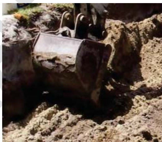
Figure 5-15. For infiltrating practices, mitigate subsoil compaction by ripping grade to a depth of 12 inches.
