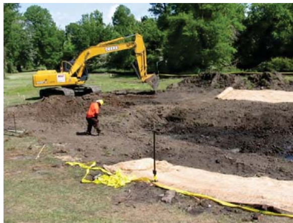
Figure 5-14. Heavy equipment (especially wheeled equipment) should be operated outside the excavated area to prevent compaction.
