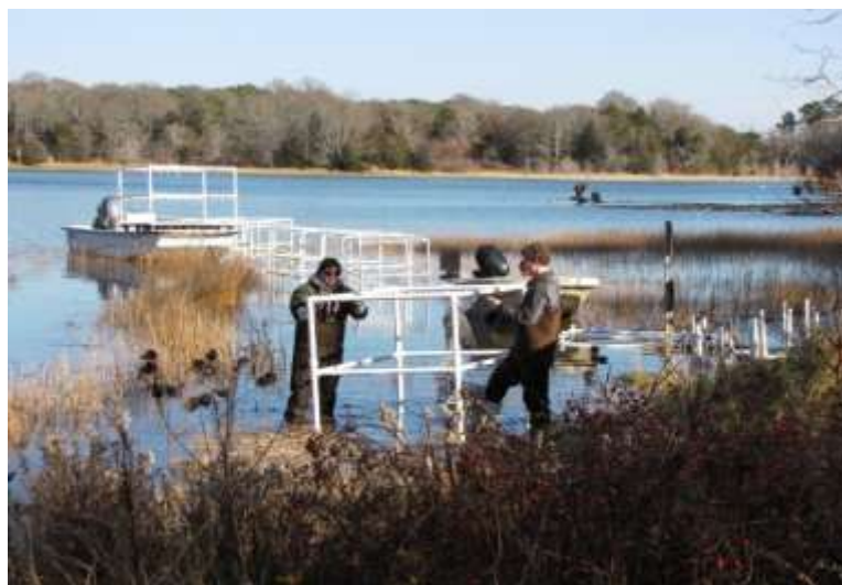
Figure 23 - Staging of Overwintering System for Installation
