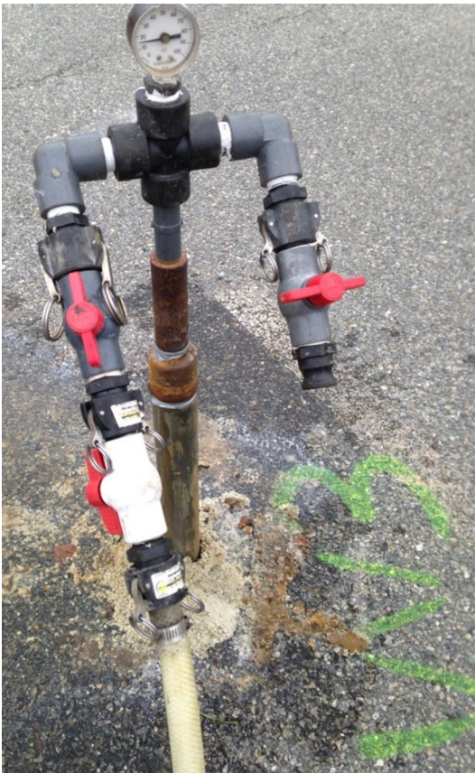
Figure 6: Direct Push Injection Point During Injection (Left) and After (Right)
