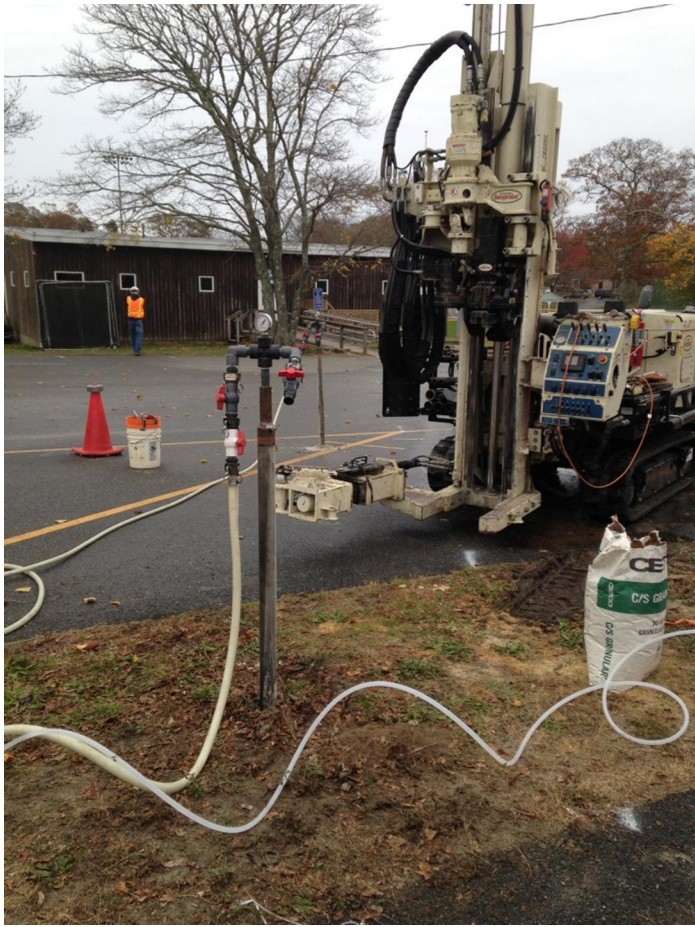
Figure 4: Direct-Push Injection Point and Geoprobe
