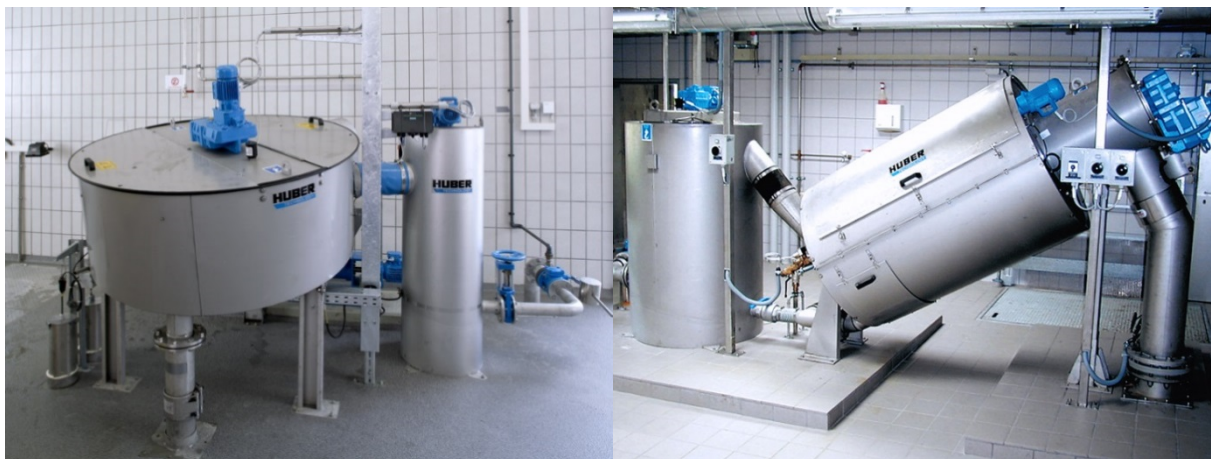
Figure 5: Example of Screw Thickener (Huber Technology, Inc.)
