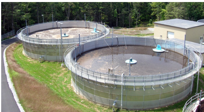
Figure 2: Sequencing Batch Reactors (Aqua-Aerobic Systems, Inc.)
