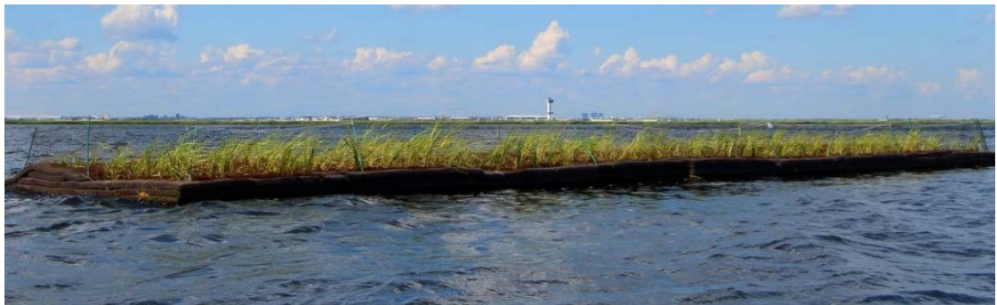
Jamaica Bay Floating Wetland Wave Attenuator
