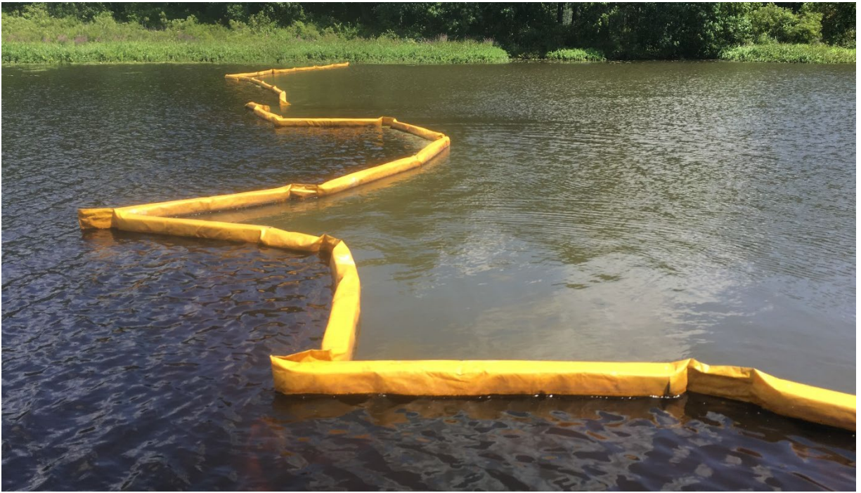
Photo 3: View of installed siltation barrier with the barrier's flotation visible.
