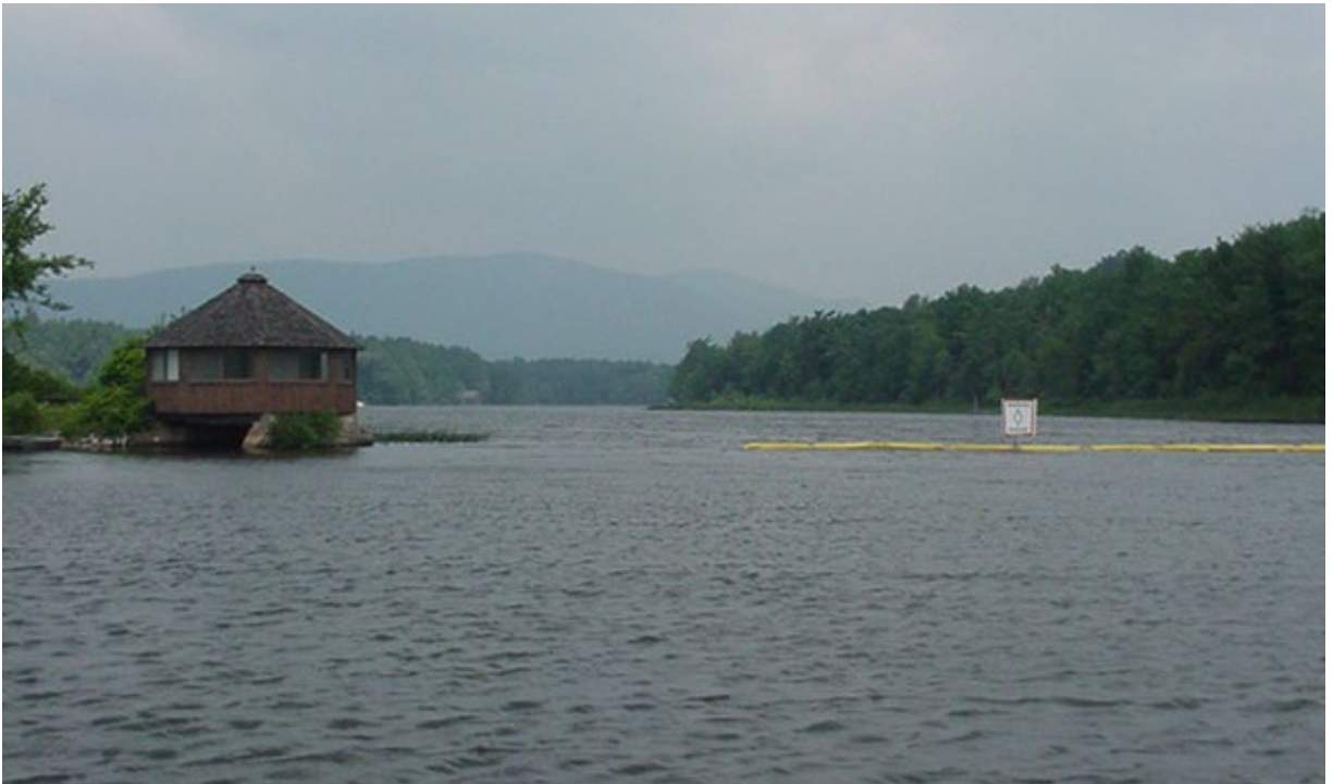
Photo 2: View of installed siltation barrier with the barrier's floatation visible.
