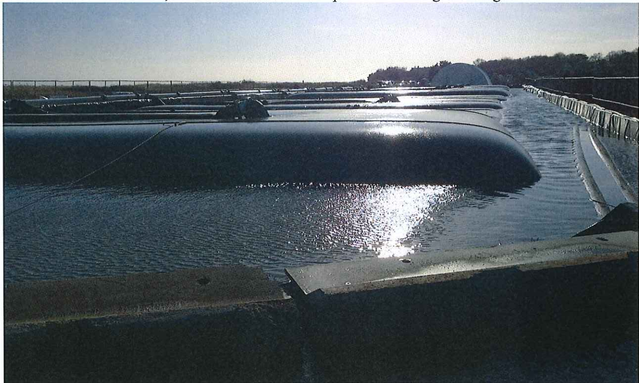
Geotubes, containment berm and process building in background
