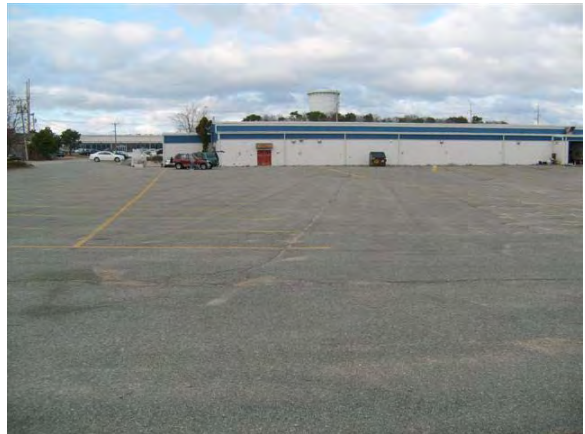
Figure 119: Charles Moore Arena Parking Area
