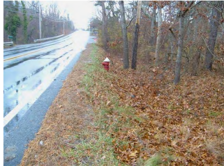
Existing Condition – East Side
