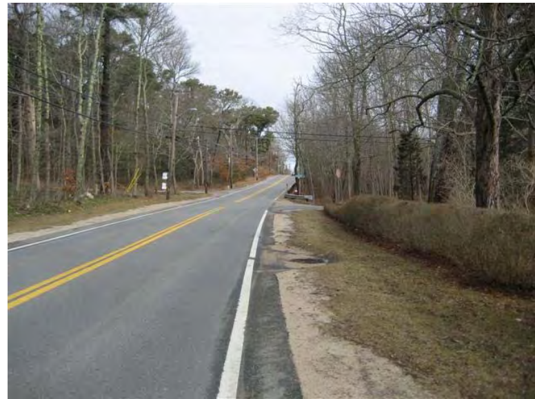
Existing Condition – East Side
