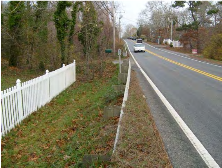
Existing Condition – West Side
