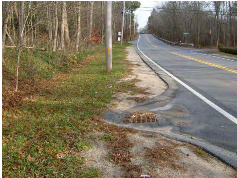
Existing Condition – West Side
