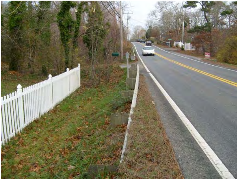
Existing Condition – West Side
