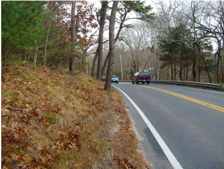
Existing Condition – West Side
