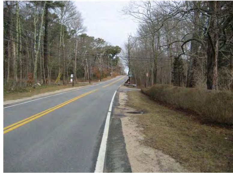
Existing Condition – East Side
