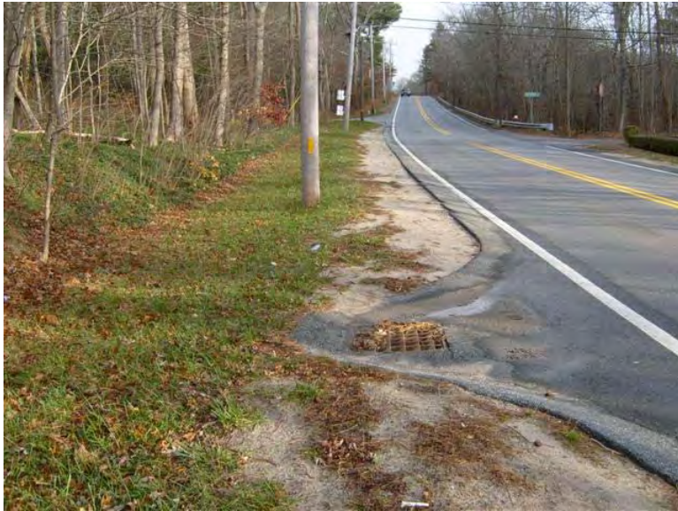
Existing Condition – West Side
