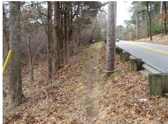
Figure 31: Existing Worn Walking Path Along Route 28 Corridor
