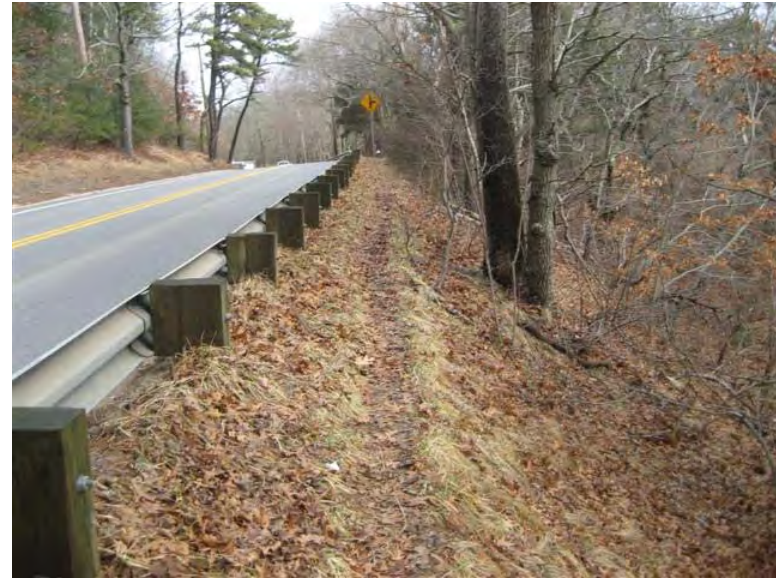
Existing Condition – East Side
