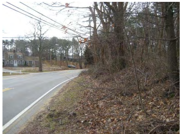
Figure 37: Sight Distance Constraint West Side of Route 28 at Monument Road
