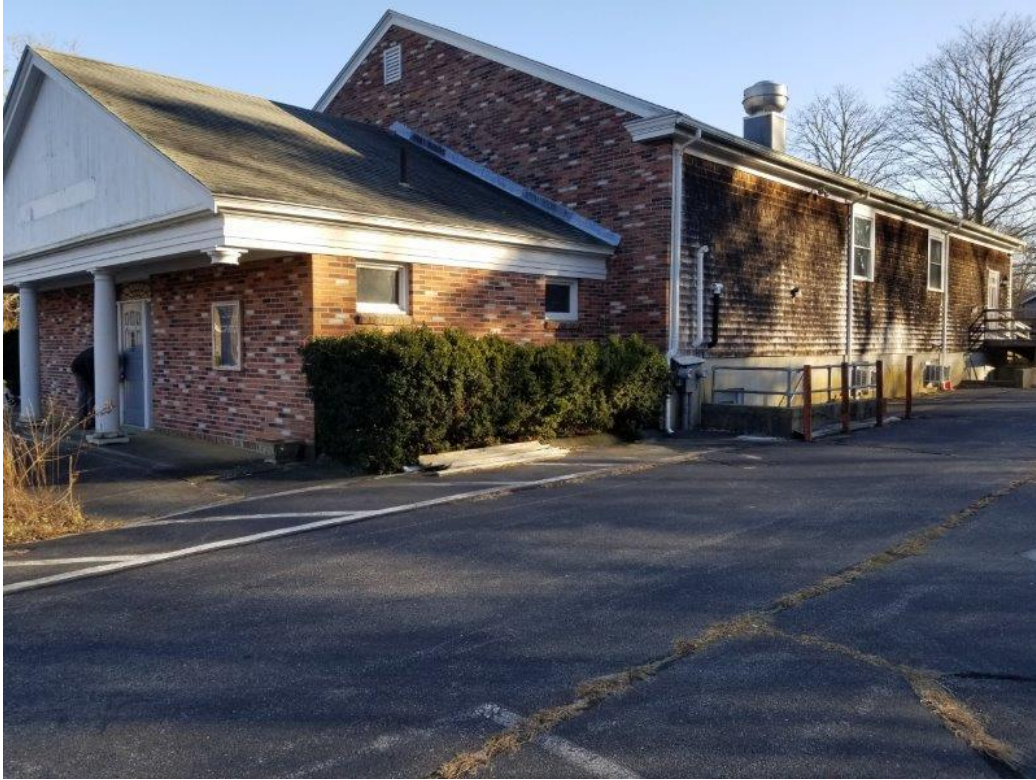
Front and west side of building
