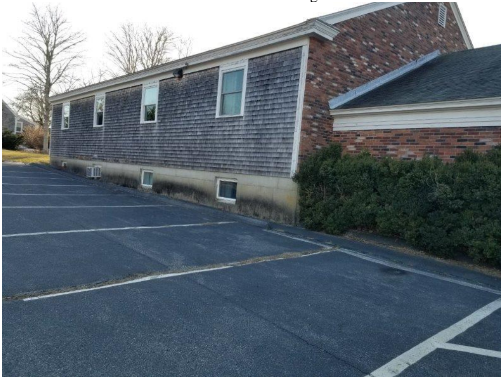
East side of building
