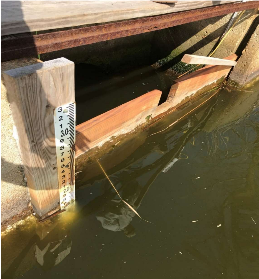
Figure III-1. Notched Board at Cedar Pond Outlet. After reviewing 2018 water levels at the outlet, Town, MassDMF, and CSP/SMASST staff agreed that the boards at the outlet could have a notch in the upper board to facilitate fish passage while also trying to limit the volume of high tides reaching Cedar Pond. Subsequent water level monitoring in 2019 showed that once a notch was added, salinity levels increased at the same rate as in 2018 when the boards were lowered. 2020 monitoring suggested that the elevation of the bottom of the notch could be increased while also attaining similar frequency of water levels meeting the Fishway Plan goals. Notch elevations are adjusted according to Fishway Plan goals for 6 inches of water over the notch bottom in the spring for spawning herring immigration (March 15 to June 30) and 2 inches of water over the notch bottom in mid/late summer to allow young of the year emigration (July 1 to November 15). No herring had been observed during more than 81 visits from 2018 through 2021, but use of fyke nets by Town and MassDMF in March/April 2022 trapped and released 30 alewife. Herring in the Cedar Pond Creek is one indication of improving water quality conditions in Cedar Pond.
